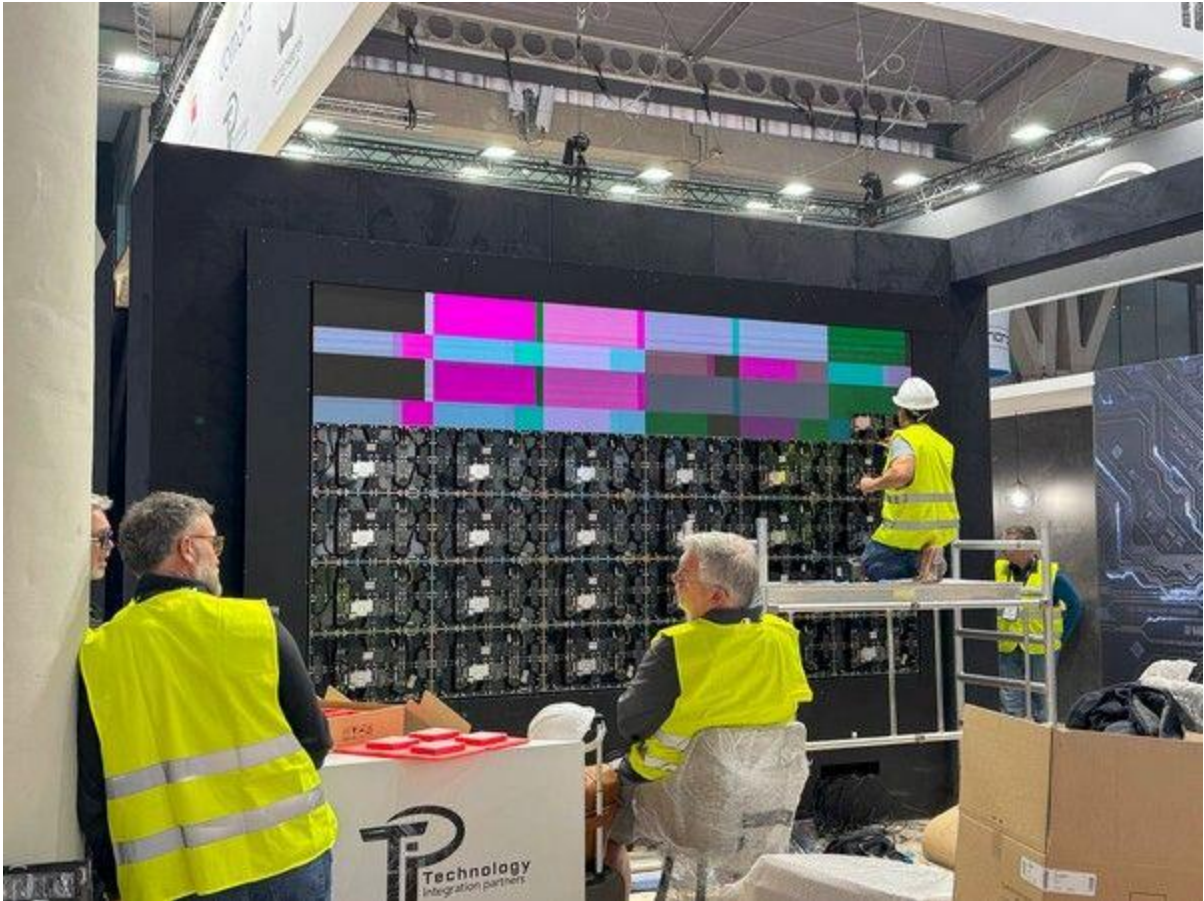
167" Barco Video Wall with Envy Extreme MK2 under construction
